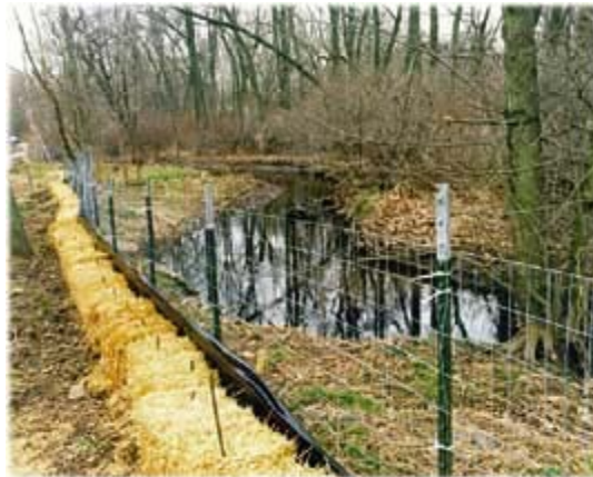
Reinforced silt fence.
