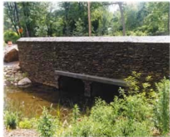
After: expanded culvert with reconstructed headwall and landscaping
