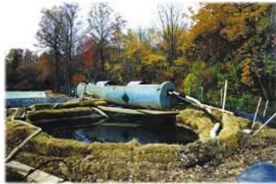
Portable sediment tank with sediment trap
